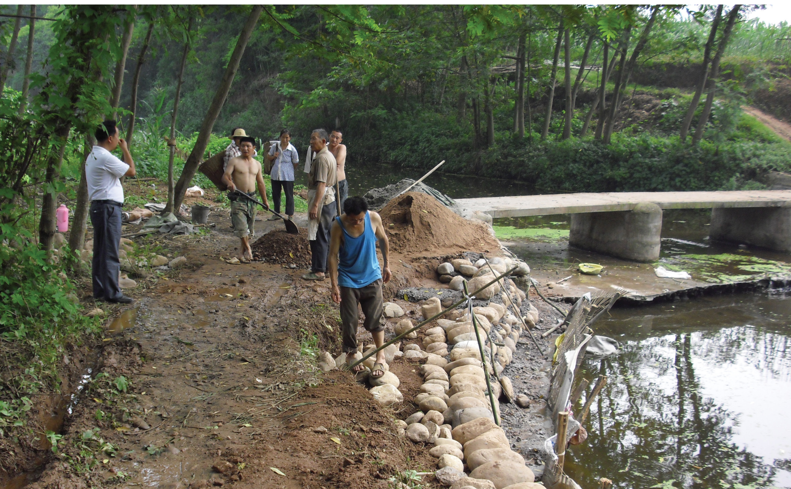
Picture 10: River bank and irrigation system maintenance with Chengdu PB village funds Source: PB Chengdu, 2014
